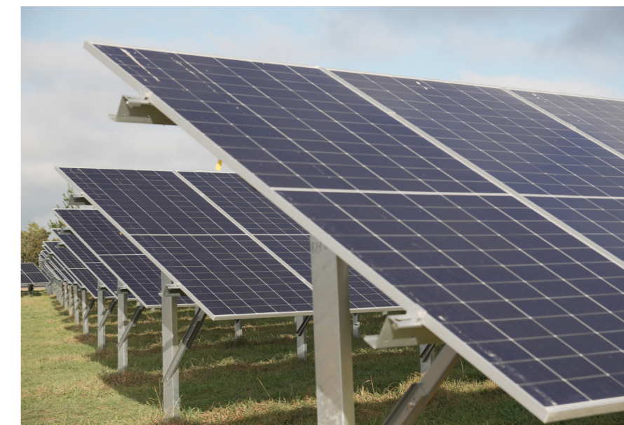
Thongcaster Road solar farm, site blessing and ground breaking.
