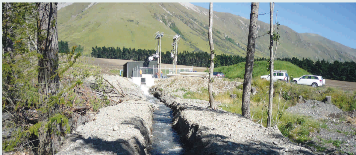
Cleardale Hydro Scheme Power House
