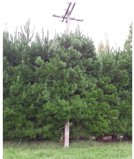
Examples of unsafe power poles and lines.
